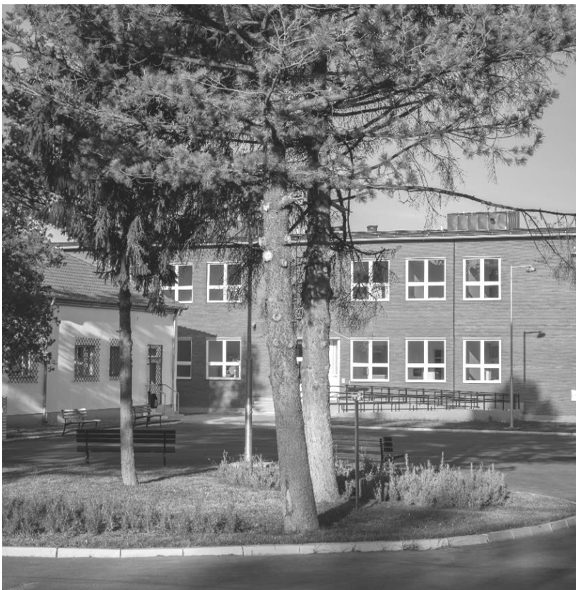
Photograph 3: A look on the new accommodation building in the Correctional Institution for Women in Požarevac. The author of the photograph: Ana Batričević. The photograph was made in 2019 with the permission of the Administration for the Execution of Criminal Sanctions, Ministry of Justice of the Republic of Serbia
