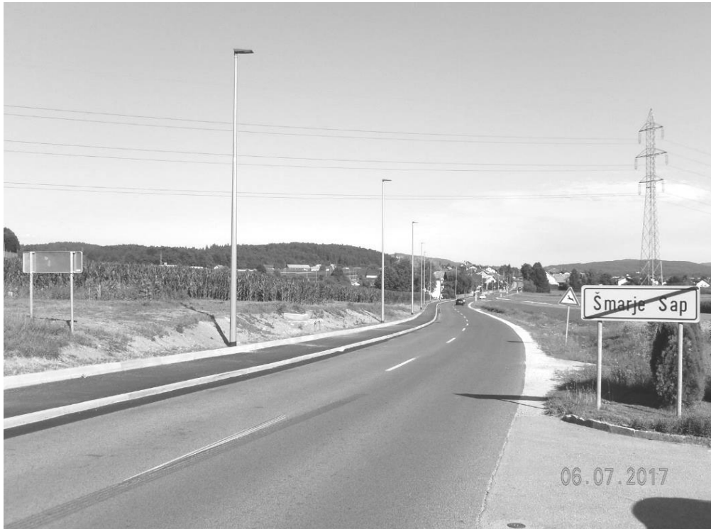
Figure 4: Passive safe poles in the 90 km/h zone - no need for a barrier.
