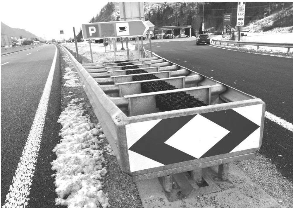
Figure 2: Crash cushion shielding the exit to the rest area.
