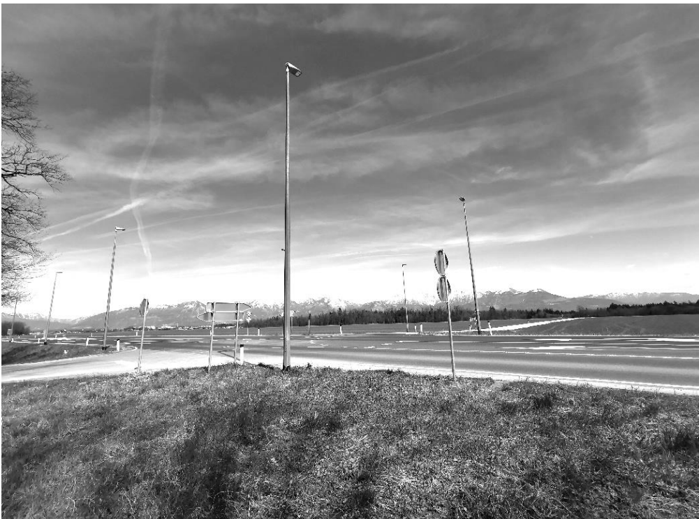
Figure 1: Roadside cleaned from hazardous objects, poles are passive safe.
